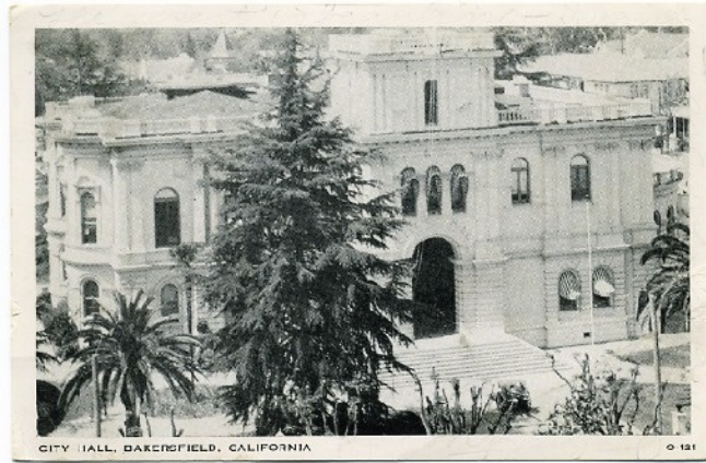
Old Kern County Courthouse, above, became Bakersfield City Hall
