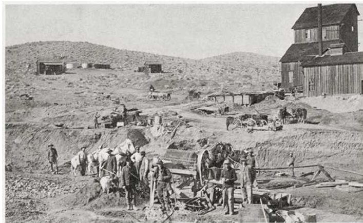
THE BALTIC MINE WITH TEN-STAMP MILL AND CABINS IN THE BACKGROUND; PLACERING OPERATIONS IN THE FOREGROUND
