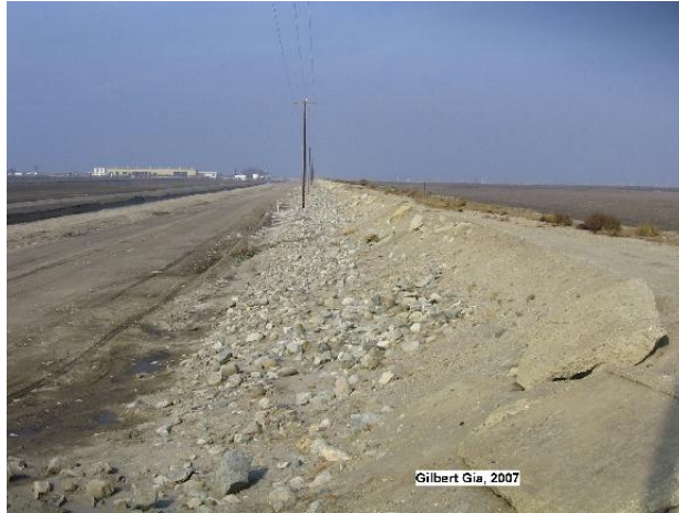
Levee at Buena Vista Lake, 2007
